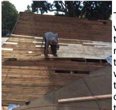
To start with we had to patch the roof where the water would just gush in then rip up the wood floors next to the windows, replace the floor joist, rebuild the wall, all
